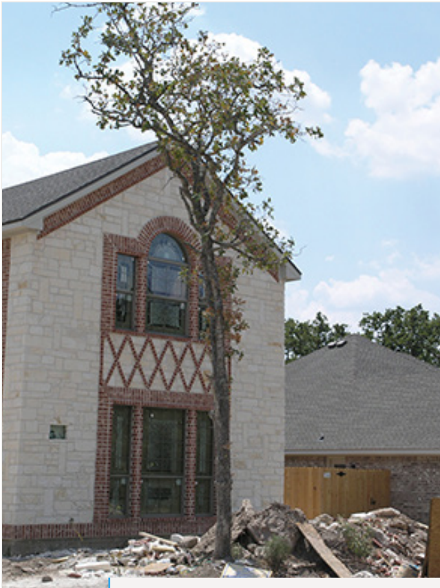
Figure 6. Typical site disruptions during home construction. Source: David N. Appel
